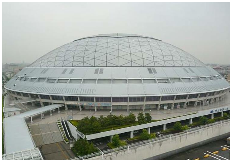
Figure 1. Nagoya Dome Sports Complex 1997, Nagoya, Japan. Dome with a diameter of 188 m made of steel pipes with a diameter of 65 cm.
